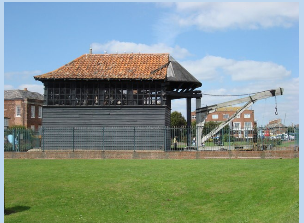
Harwich has a 17th century dockyard treadmill crane.
